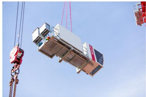
Assembly of the cabin platform with WOLFF Cab and control cabinet.
