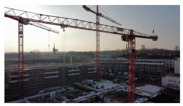
The low assembly height of the flat top WOLFF Clear crane keeps the crane concept low and thus profitable. The entire construction site 0f 15.600 m2 is covered with only three cranes.
