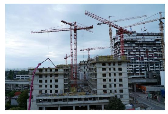
Crane to crane: the cranes from the neighboring Marina Tower construction site protrude into the Donaumarina residential complex and thus had to be taken into consideration in the planning process for the crane concept.
