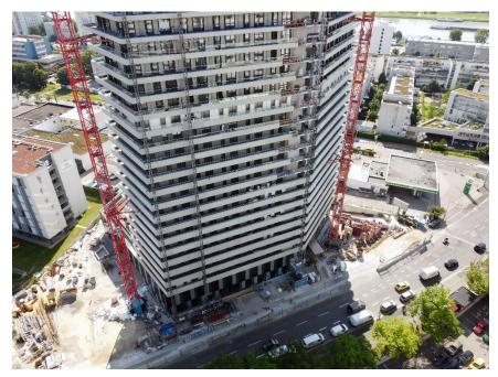
Despite their impressive height, the cranes manage with only two tie-downs each. This brings economic advantages and the construction process is disturbed as little as possible.
