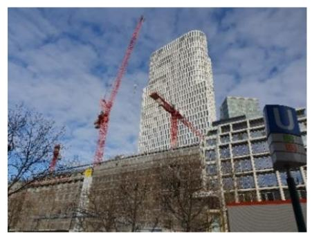
The WOLFF 180 B dismantled the two supporting WOLFF clear cranes 5020.8 and 6015.8 on the extremely space restricted job site in Berlin.
