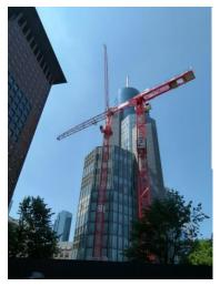
The almost vertical position of the jib and the short counterjib of the WOLFF 355 B luffing crane as well as the flat-top construction of the 6031.8 clear make the WOLFFs an ideal choice for large-scale inner-city construction sites.
