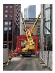
Assembly of the WOLFF Cityportal, with internal dimension of 6.2 x 6.2 meters and a clearance height of 4.5 meters, to ensures the free flow of traffic.
