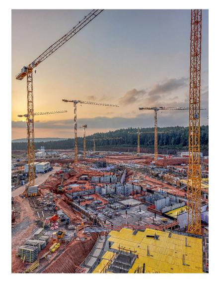
Due to the very deep base layers, some of the crane foundations had to be integrated into the buildings and will remain in the ground once the construction work is complete. Temporary shoring around the tower sections enables the crane to be completely dismantled even after the working area has been backfilled.
